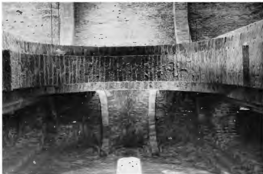
FIGURE 8. Sant Vicenç de Cardona, intrados of nave arcade, with vaults to nave and north aisle (Peter Reed).
